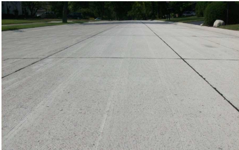
Example of a diamond-ground street
