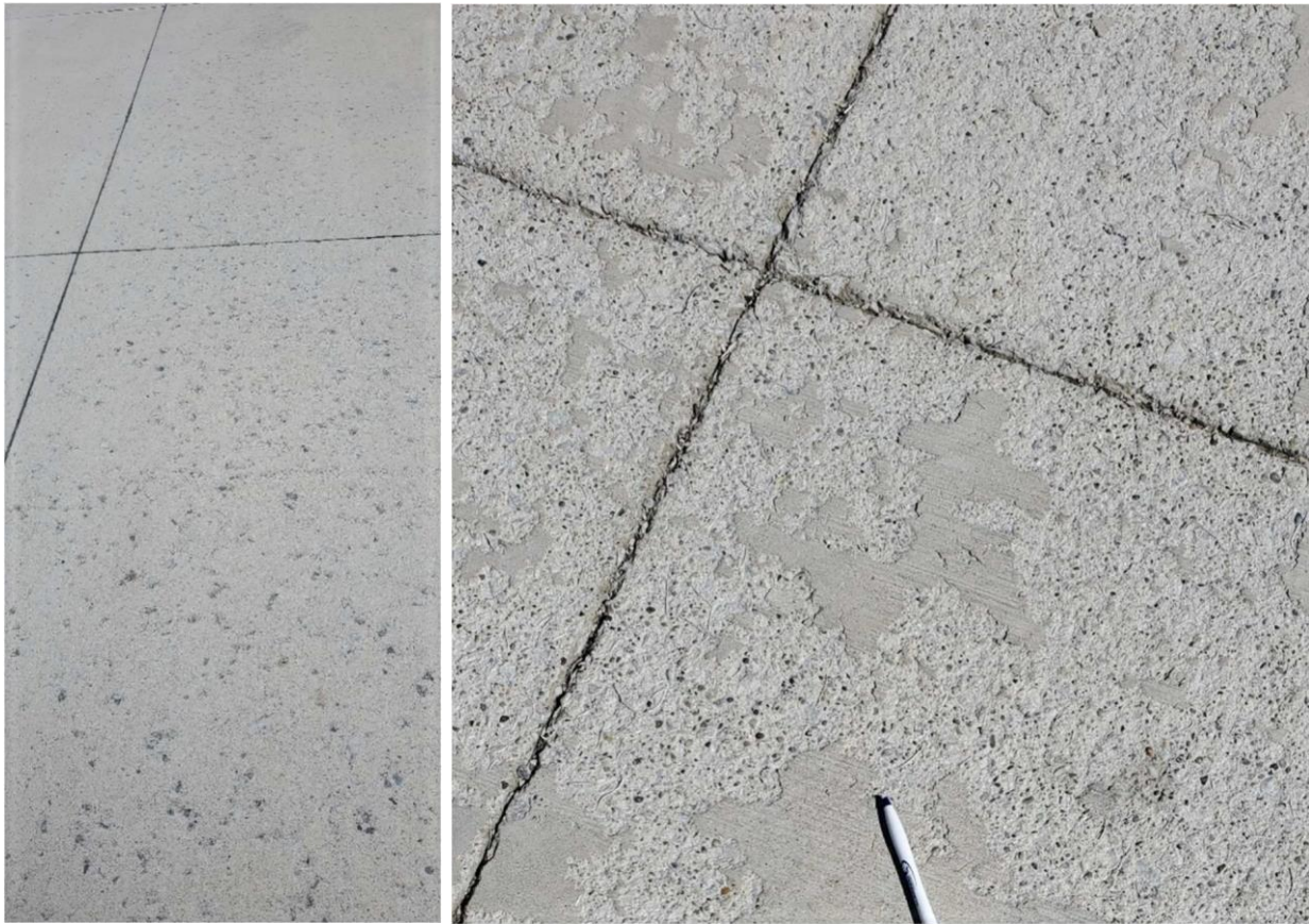
Examples of scaling (left, light severity, sometimes called mortar flaking; and right, medium severity)
