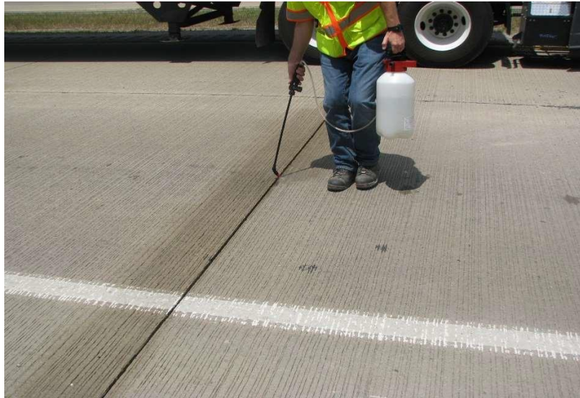
Application of a penetrating sealer to concrete
