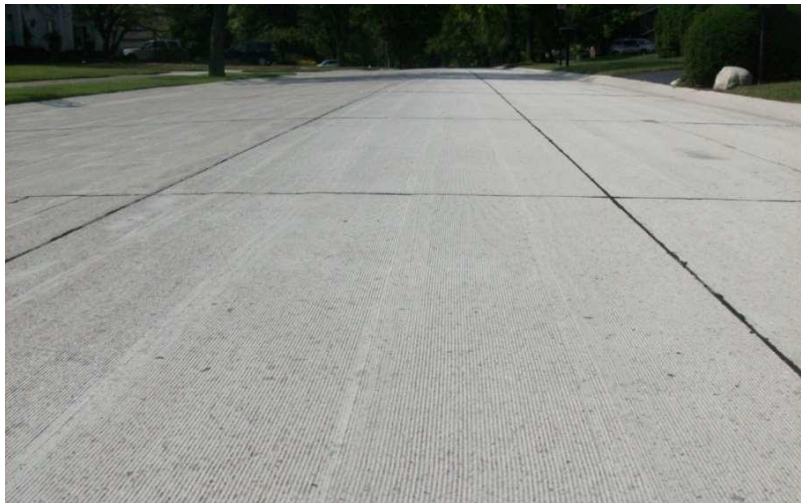
Example of a diamond-ground street
