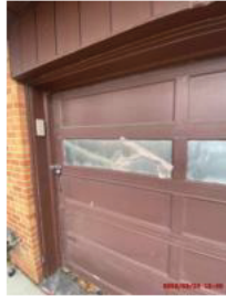
Cracked/damaged garage window.
