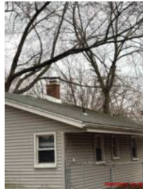
Newer roof no visible interior water damage
