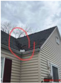
Valley of the roof has a leak
