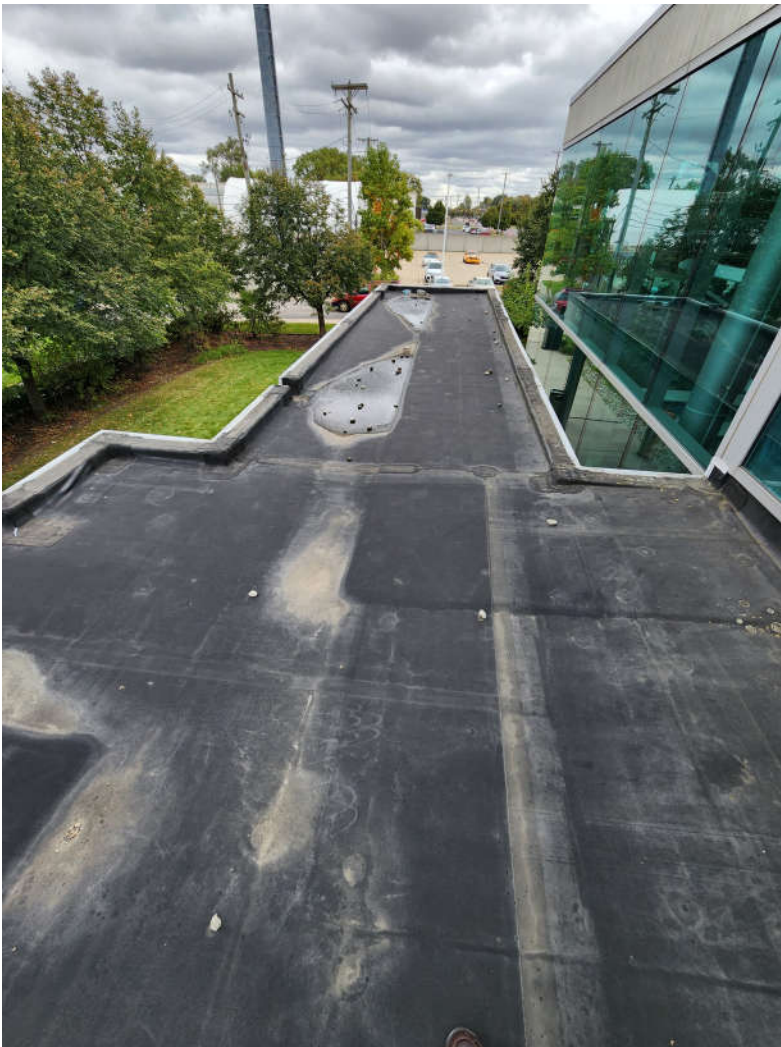
Overview of the canopy above the entrance doors looking east.
