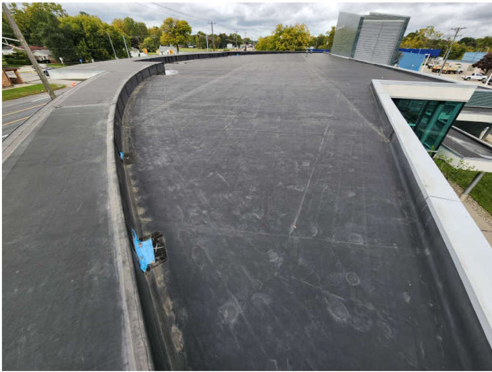
Overview of the main roof from the east looking west.
