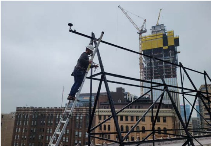
Installing the RTK/GNSS base station that was used to collect the data for the project.
