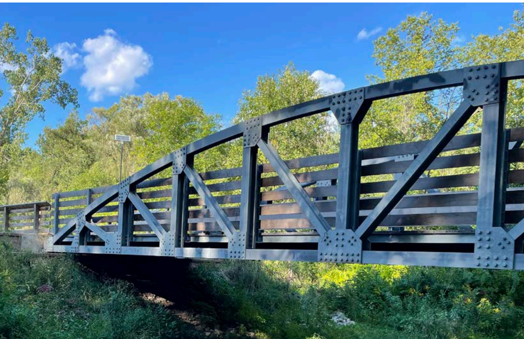
Paint Creek Trail Bridge, Rochester, MI
