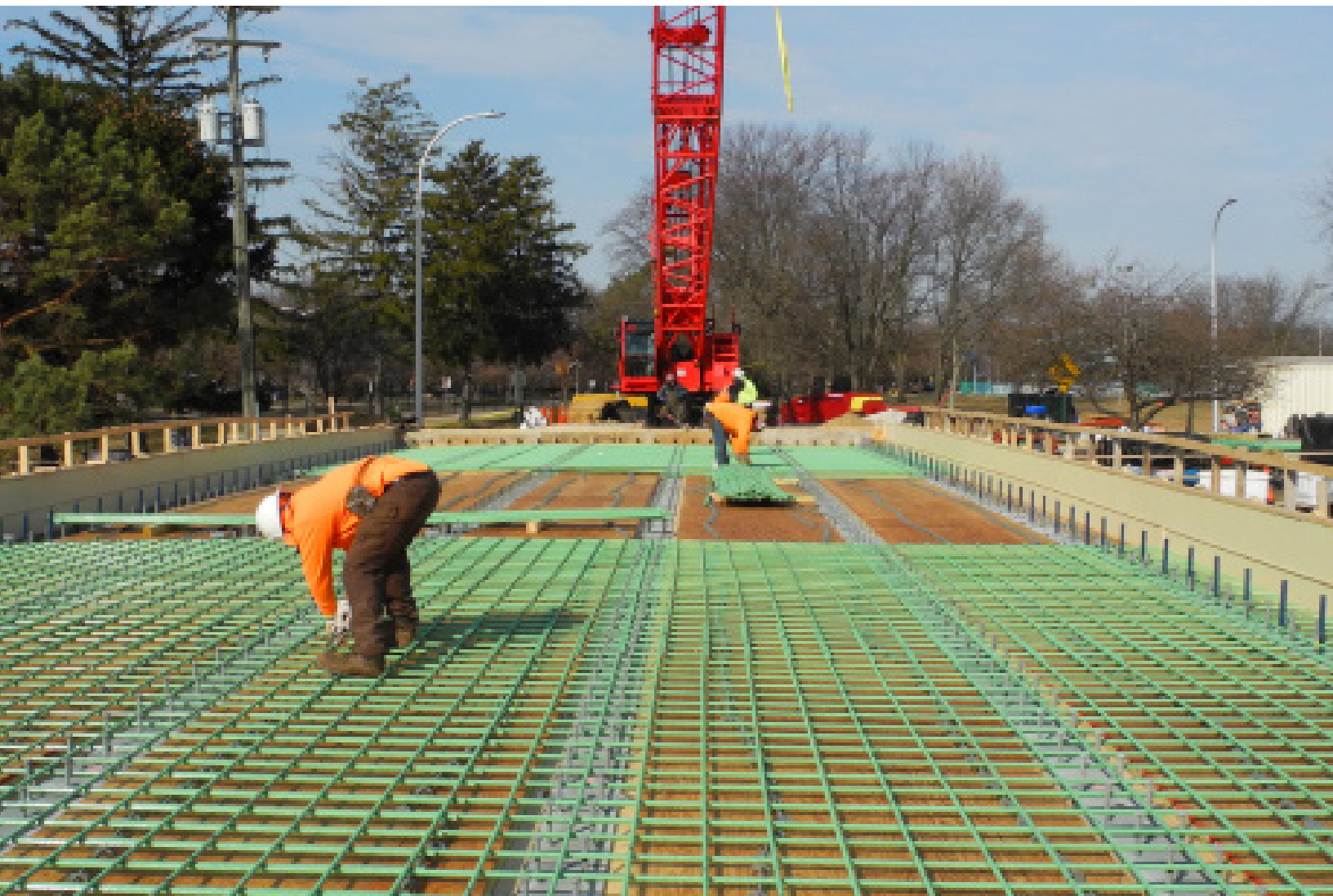
Rebar Installation on Deck of Lake Front Park Bridge, Grosse Pointe Woods, MI
