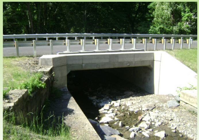
Strossertown Bridge Replacement
