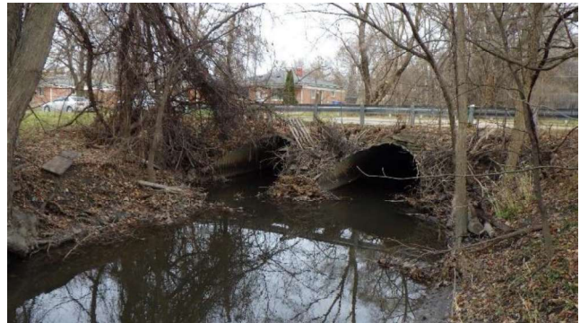
Polk Street over Ecorse Creek
