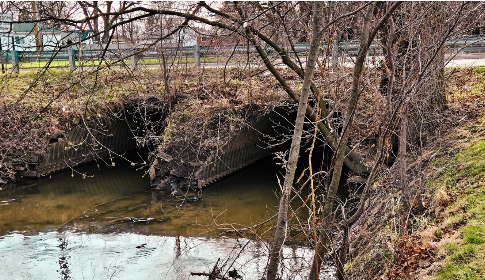
Bridge Culverts Under Polk Street at Ecorse Creek
