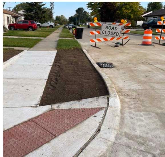
Northview Project Under Construction
