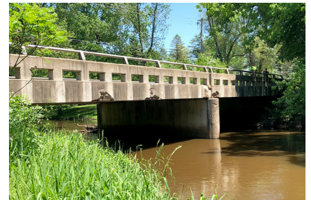
Herbison Road over Looking Glass River
