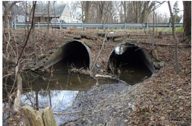
Figure 1: Hipp Street over Ecorse Creek
