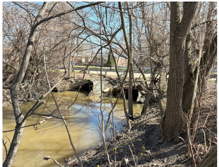
Polk Street Culverts
