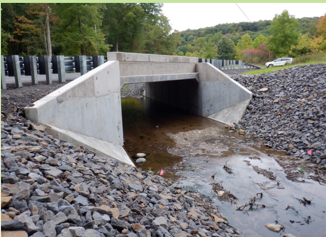
Market Street Culvert Replacement
