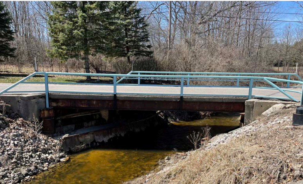
Kellie Boulevard Bridge over Bunce Creek, Marysville, MI
