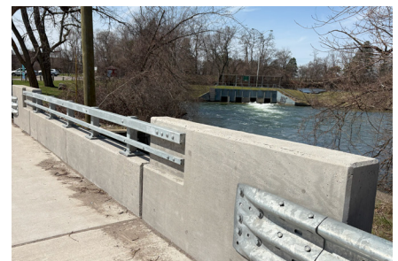
View of the new aesthetic bridge parapet
