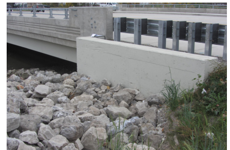
Northwest return wall and scour control riprap
