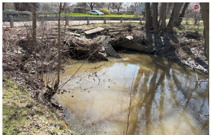
Hipp Street Culverts
