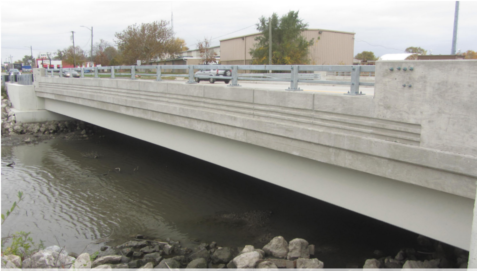
Southfield Road over Ecorse Creek elevation view
