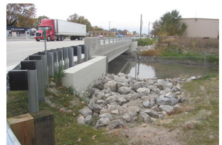
Deck surface and barrier railing
